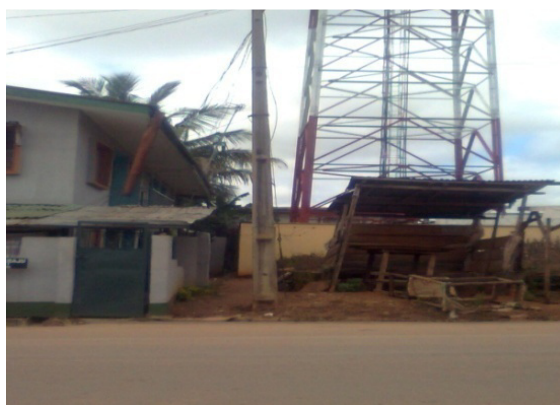
Plate 1: Glo Mast Very Close (6ft) to a Building 10m in than OtanAyegbajustreet, Alekuwodo area Osogbo
